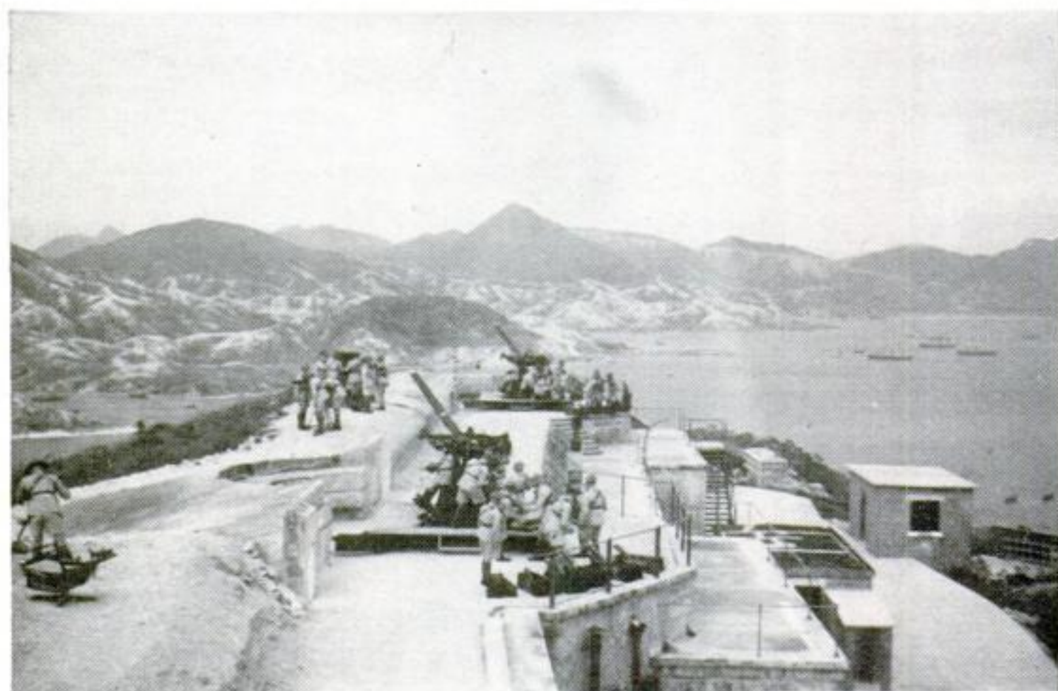
Anti-aircraft rifles bristle from the peaks of Hong Kong Island guarding harbor. Concrete gun emplacements and dugouts shown here have been greatly extended in the last year.
