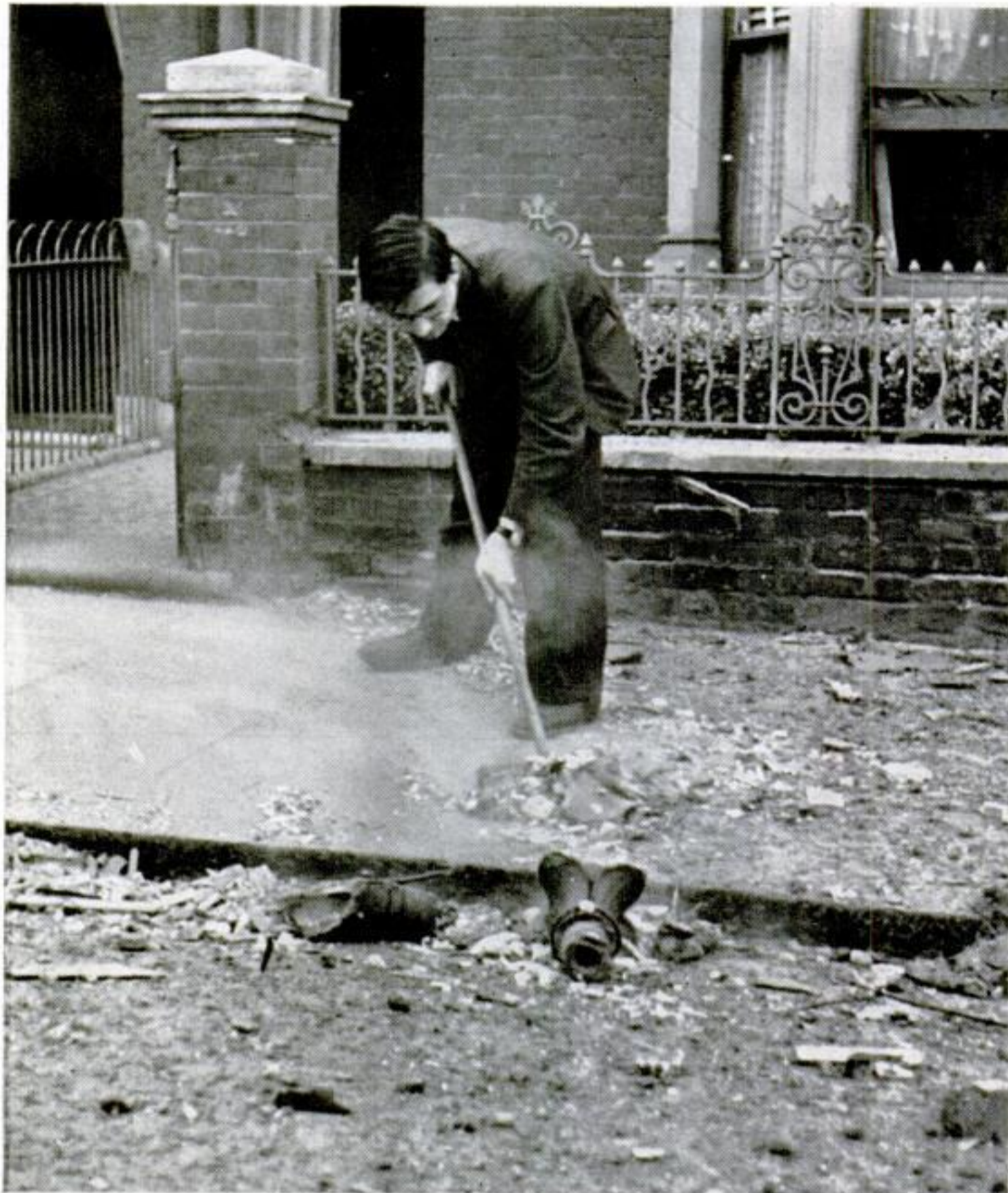
Tidying up as fast as their city is wrecked is second nature to Londoners. The all-clear siren has not yet sounded but this man is already sweeping the remains of a lamppost into the gutter. Behavior like this is what keeps London functioning through its terrible ordeal.
