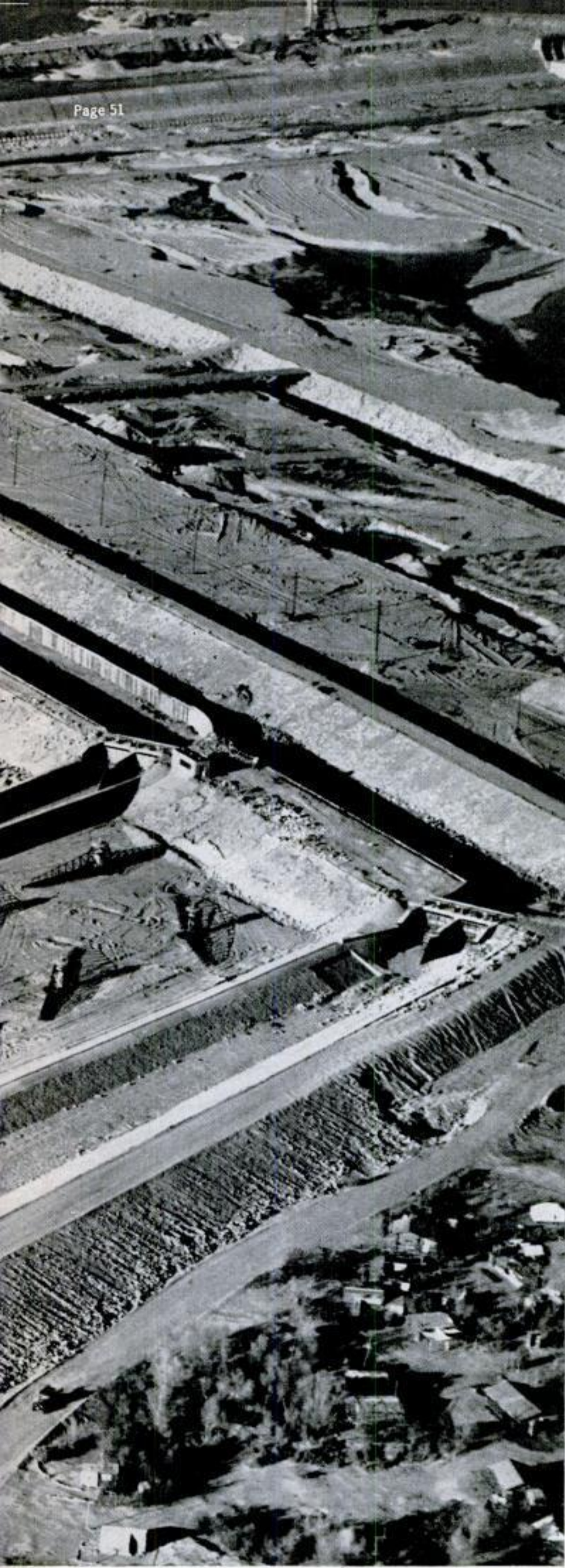
side channels, where it flows off into the canal (lower left). The ridge across the channel at left is a road which will be removed.
