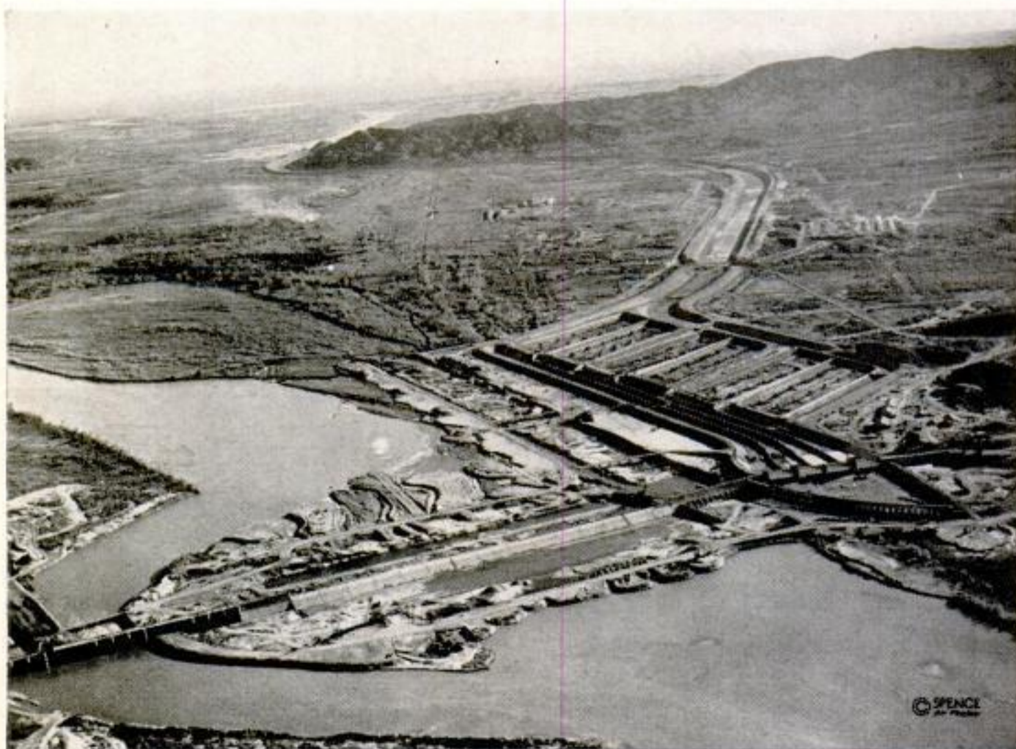
The Imperial Dam is shown here a few months before the dedication. Behind the dam are the six settling basins. Behind them, the canal curves around a mountain to the desert.
