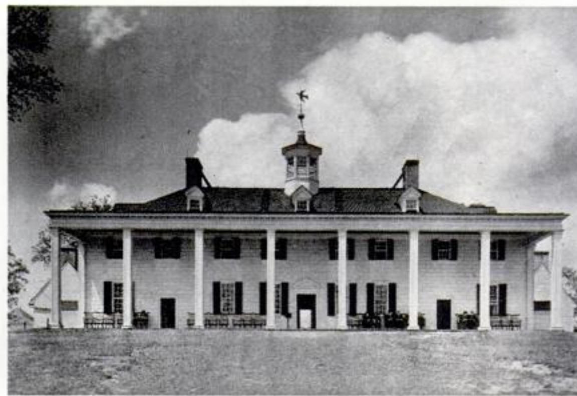
Mount Vernon , like most of the Colonial homes in America, was inspired by the architecture of Georgian England. George Washington built it of wood and extended the Georgian colonnade to a porch to suit the climate.
