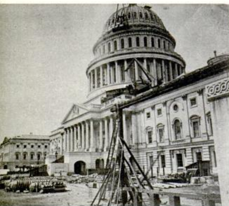
The Capitol dome , copied by almost every State in the Union, is of iron; shown before its completion in 1863.
