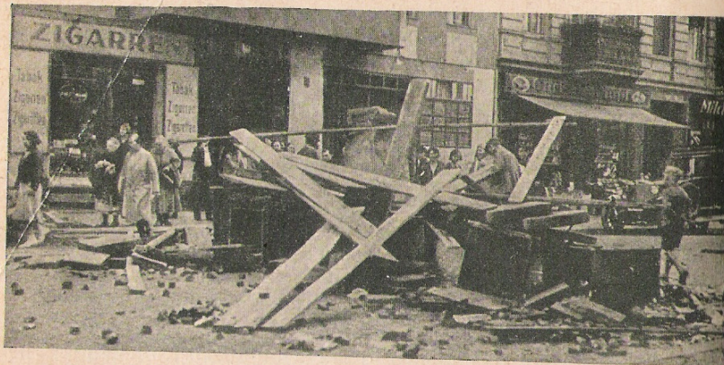
Barricade erected in the Rostocker Strasse, Moabit, Berlin, in June 1932.
